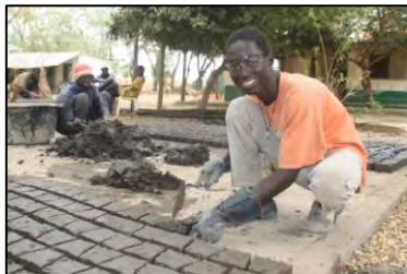
Local masons making custom bricks for the outer wall
